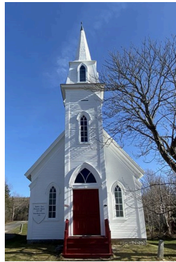
Methodist United Church 660 Hwy 1
